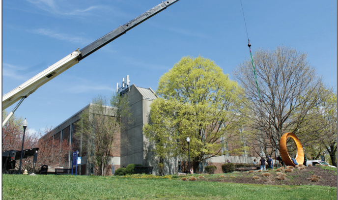
A crane used to lower the sculpture into its original location.
