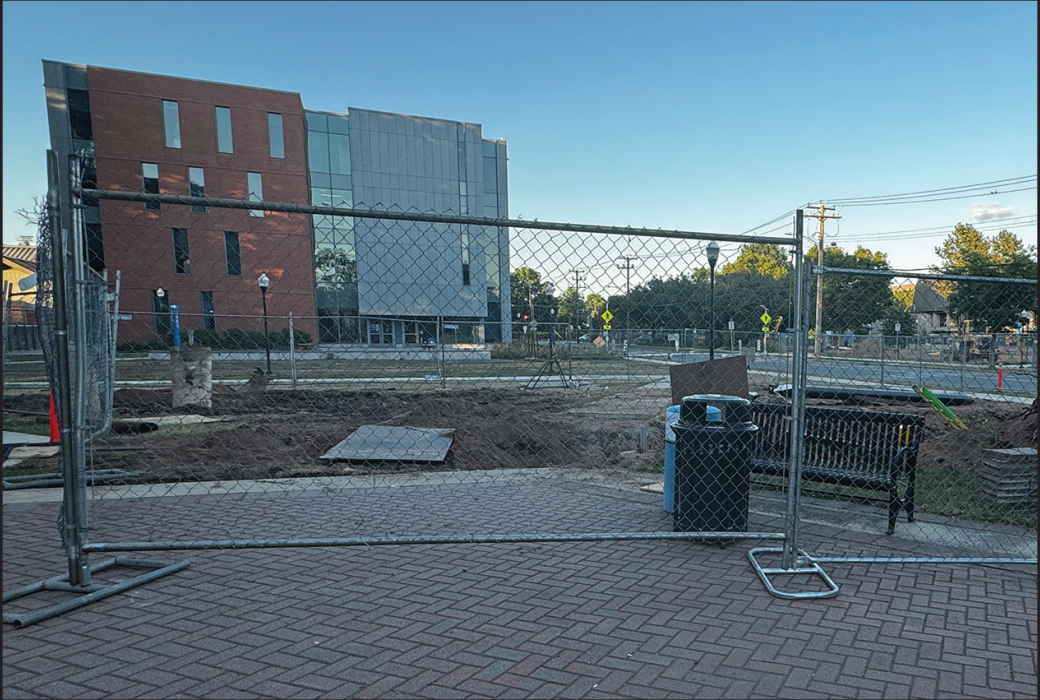
Gates blocking off the construction site in front of the School of Business on Sept. 3.
