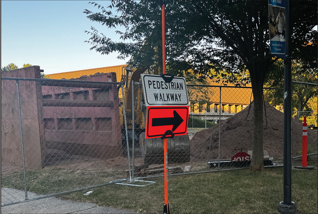
Construction site blocking off the walkway to Connecticut Hall and detouring students near the Connecticut Hall parking lot on Sept. 3.
