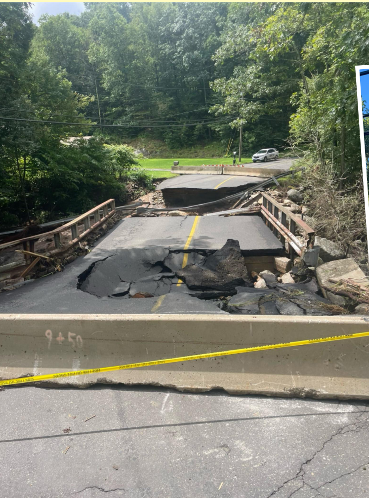
Seth Den Rd. Bridge Before
