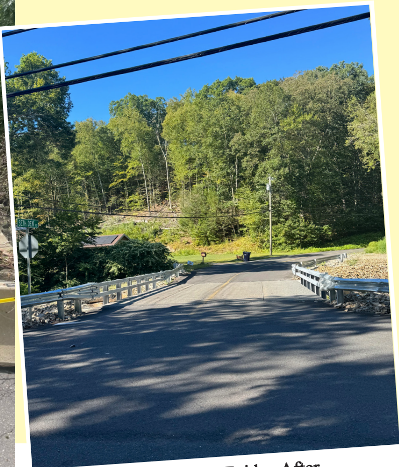
Seth Den Rd. Bridge After
